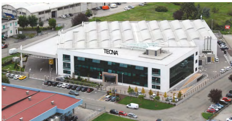
Registered office, offices, industrial production and shipments Via Meucci, 27 | Castel San Pietro Terme | GPS N44° 24' 24" - E11° 35' 13"
